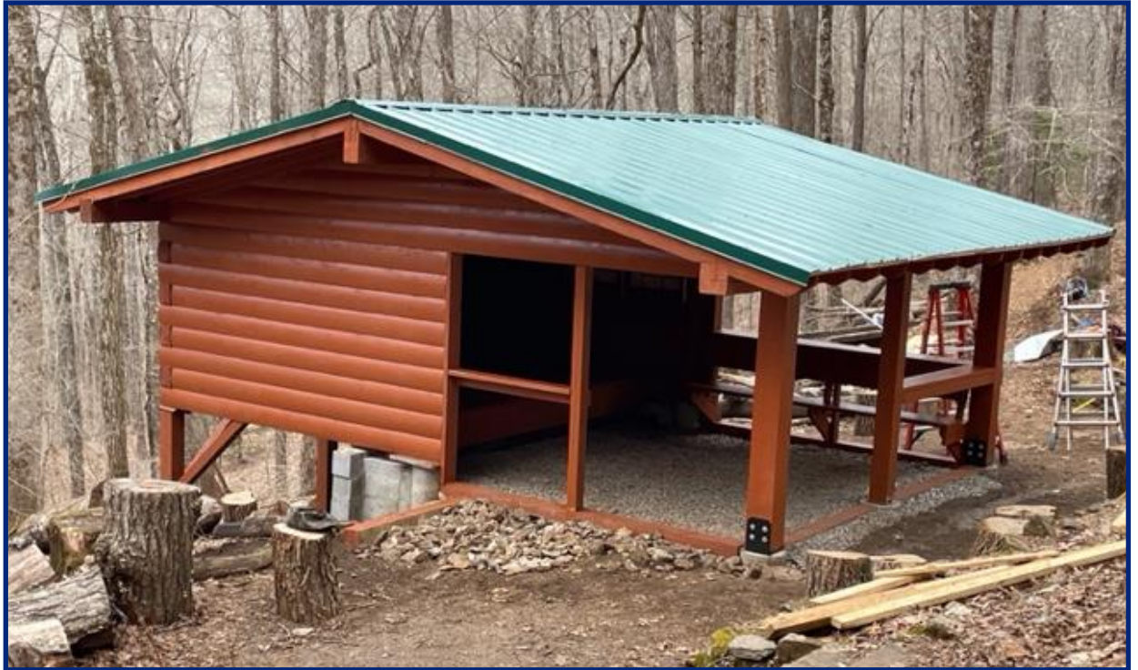
The New Rock Gap Shelter
